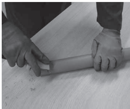
Fig. 2 Remove the outside oxide layer using a suitable scraper.
