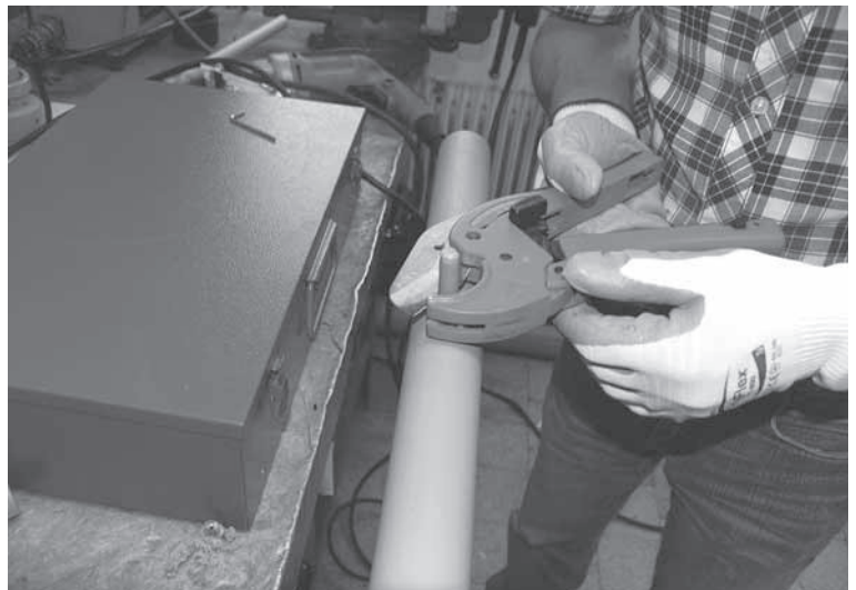
Fig. 3 After a cooling time of approx. 5 minutes, remove the protruding end of the repairing plug.
