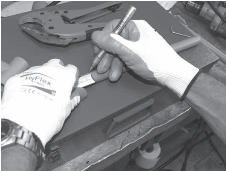
Fig. 5 Mark up the bush depth.
