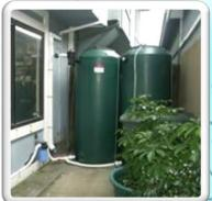
20 thru 12500 Gallon Capacity • FDA Approved Green or Black Color • UV Resistant ● FNPT Inlet/Outlet Connections ● 16" Manway Opening Access • Durable, Impact Resistant Polyethylene • Safe for Potable Water
