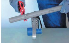
Cut the tube perpendicularly to its axis using the suitable pipe cutter.
