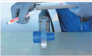
Mark the insertion depth on the pipe.
