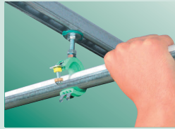
Place reinforced pipe into clamp
